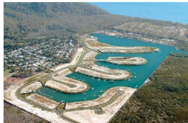
Bluewater Canal Development, Cairns.
