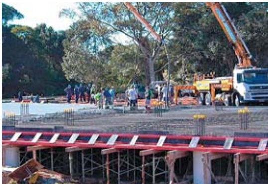
Hutchies at work on the Woolworths Maleny site.
